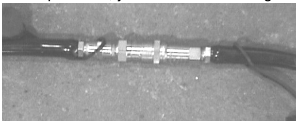
BLEEDING OF THE HYDRAULIC SYSTEM
