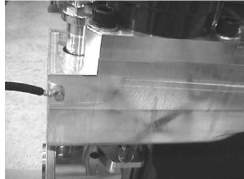
LOCATION OF GROUNDING SPIKE
